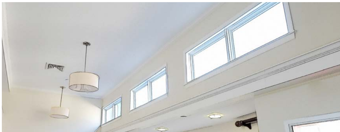
Figure 32: Clerestory lighting at White Oak Cottages. Photo Credit R.Wrublowsky, 2016. Westwood, MA. EGA Architects.
